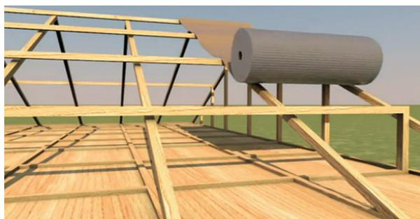
1. Roll out the Kingspan AIR-CELL® product from the ridge to gutter, over and perpendicular to the roof battens.
